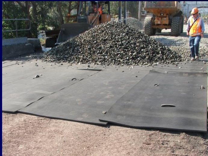
Placing of synthetic energy absorbing mats (SEAM)
